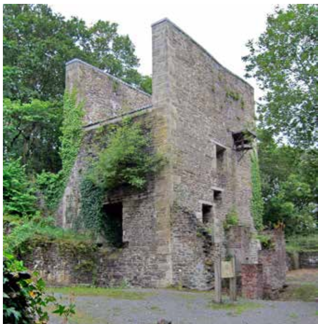
1858 pumping engine house above Lordshill shaft. Photo Tim Wellburn
